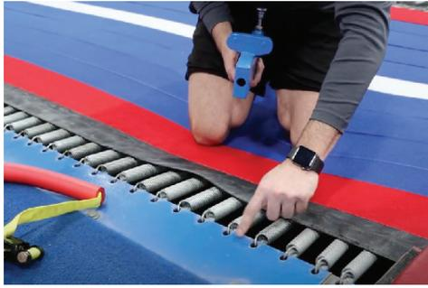
**Step 1:** Locate the area you want to place the Quick Flex Bar. Remove the padding to locate the springs.
