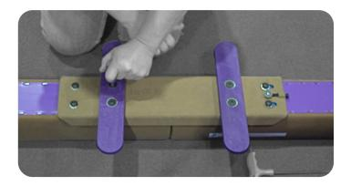
8. Tighten the adjustment screw with the 5mm Hex Wrench (H) to pull the beams together. Stop tightening when the beams stop moving together or when the end of one beam begins to lift off of the floor.
